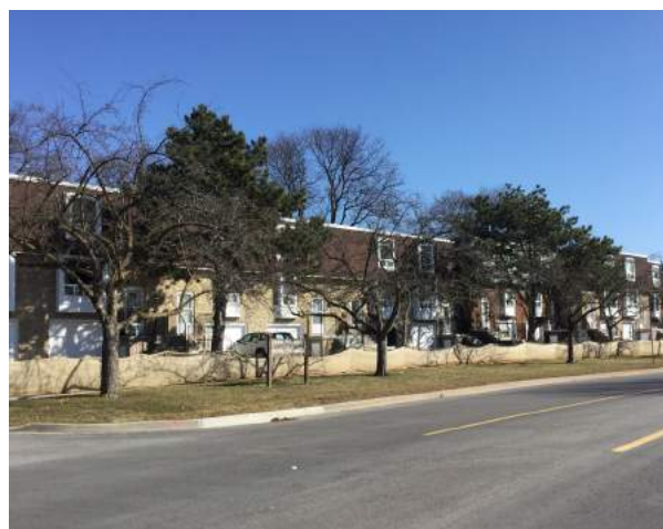
Townhouse dwellings, north side of Royal Orchard Boulevard
